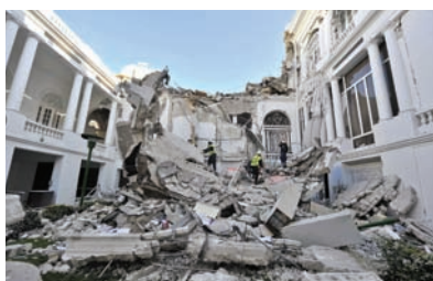
Figure 9.1 Presidential palace damaged during the 2010 Indian earthquake. (Photo by Lisa Accetta/AFP/Getty Images)
